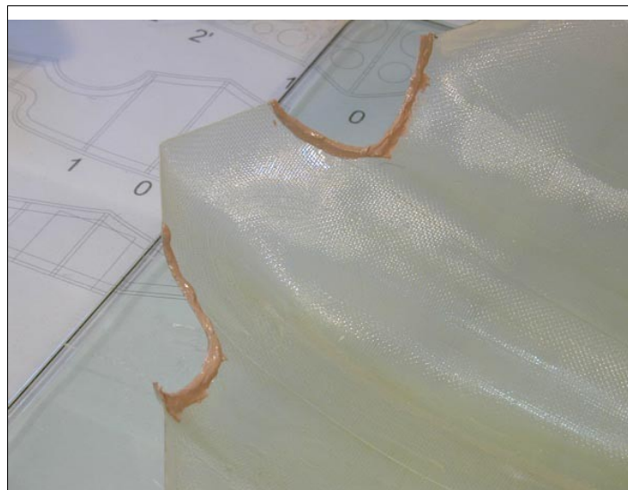
Figure 14: Applying filler to the intake area
