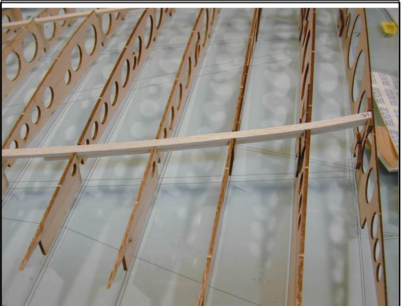
Figure 20: Installing the rear laminated spar
